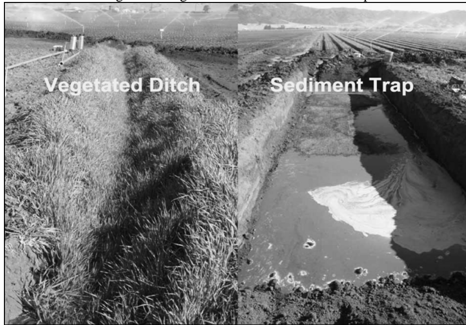
Figure 4. Vegetated Ditch and Sediment Trap
