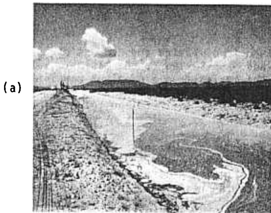
Fig. 3. Supply channel sequence during irrigation, (a) filling after water had been checked; (b) water level rising, about to enter furrows; (c) furrows being irrigated; and (d) after check gate removed and water being conveyed to a lower-lying basin. Water is still draining back out of furrows into channel.
